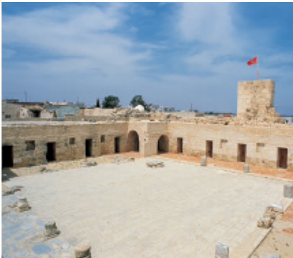
The Ribat, interior courtyard, Lemta.
