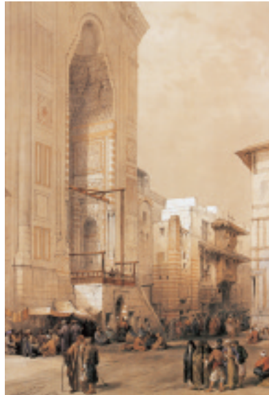
Mosque and Madrasa of Sultan Hassan, entrance, Cairo (D. Roberts, 1996, courtesy of the American University of Cairo).
