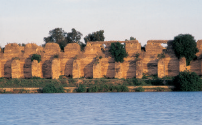
Basin of the Norias, enclosure of the ancient silos reinforced with buttresses, Meknès.
