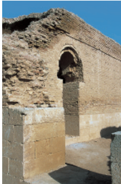
Qasr al-Mushatta, view of the brick wall at the entrance, al-Badiya.
