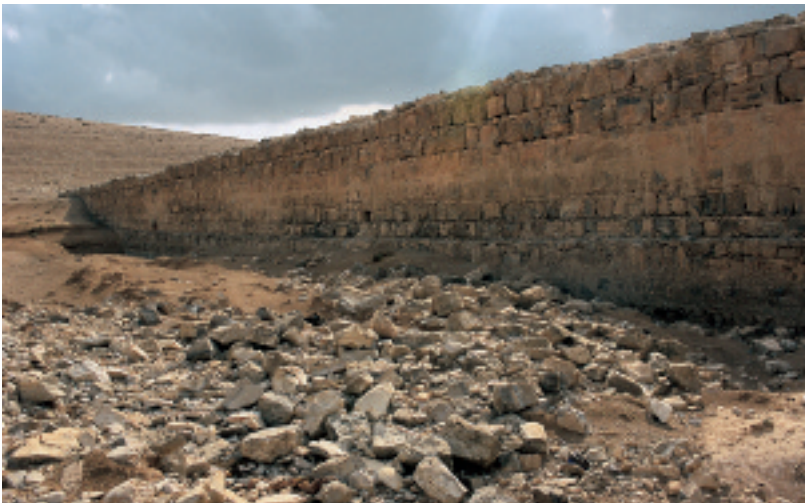
South-East Dam, al-Qanatir.
