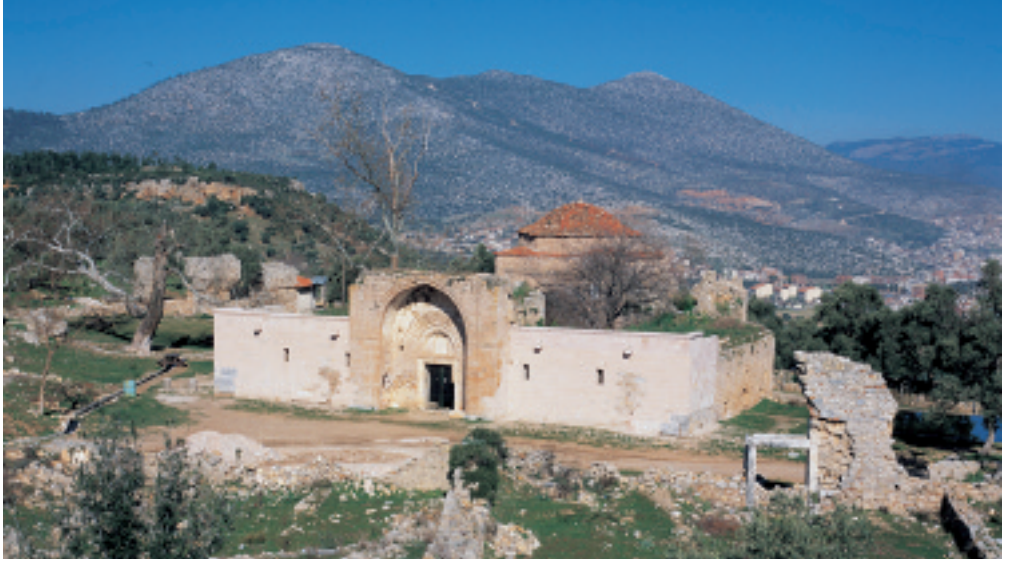
Ahmet Gazi madrasa, Entrance facade, 1375, Ahmet Gazi, Beçin.
